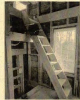
Steps to Engine Room
