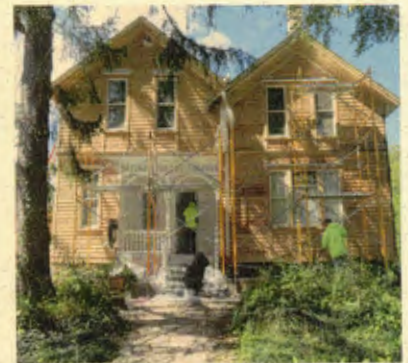
Mill House Painting in Progress
